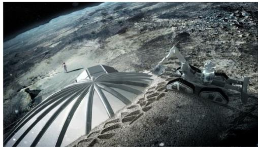
*Figure 7: Concept showing lunar rover printing over inflatable dome [9]*
